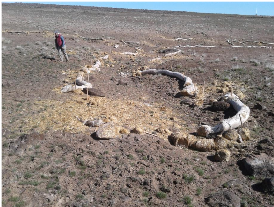
Figure 18. Straw wattles on the margins of shallow gullies on burned area on Pumhouse Road. Wattles have been partially destroyed by elk. Also, note the scant, late winter vegetation in the burned area. Source: Author photo, March 2024.
