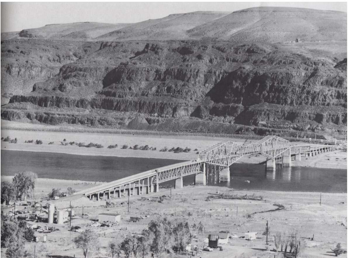
Figure 31. View east of first Vantage Bridge located at the mouth of Rocky Coulee. Completion of this bridge in 1927 eliminated the need for the Vantage ferry. In 1940, it became a key link in the U.S. Department of Defense' establishment of US 10 as Washington state's primary military route. Source: Ruby and Brown (1974, p. 101).
