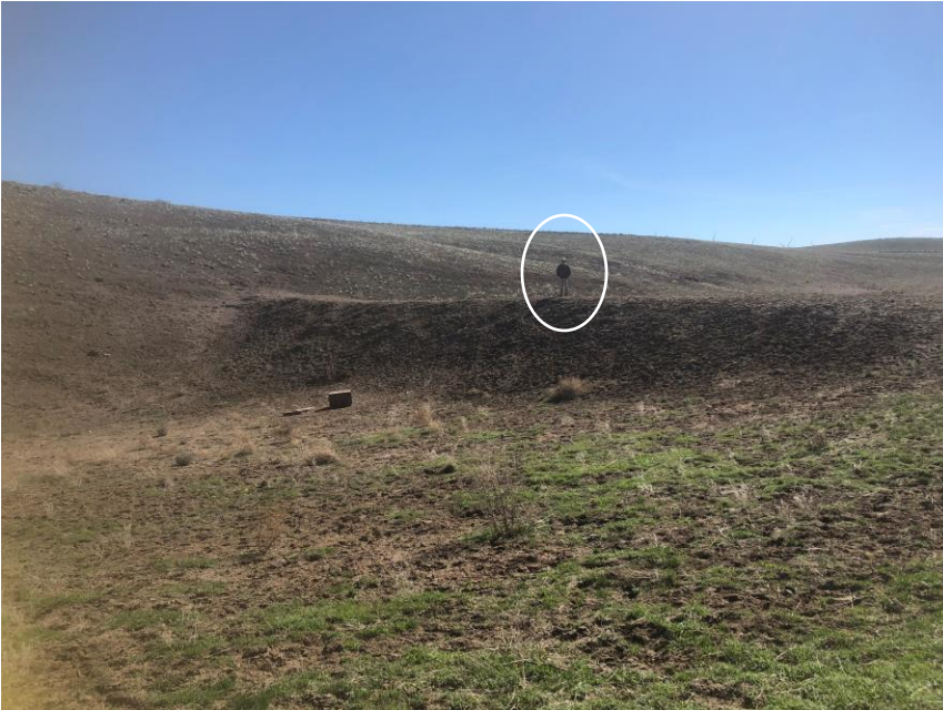
Figure 14. On-the-ground view of the downstream side of the soil-saving dam in the headwaters of Rocky Coulee. Author standing atop dam for scale. Source: Nancy Lillquist, 03/2024.
