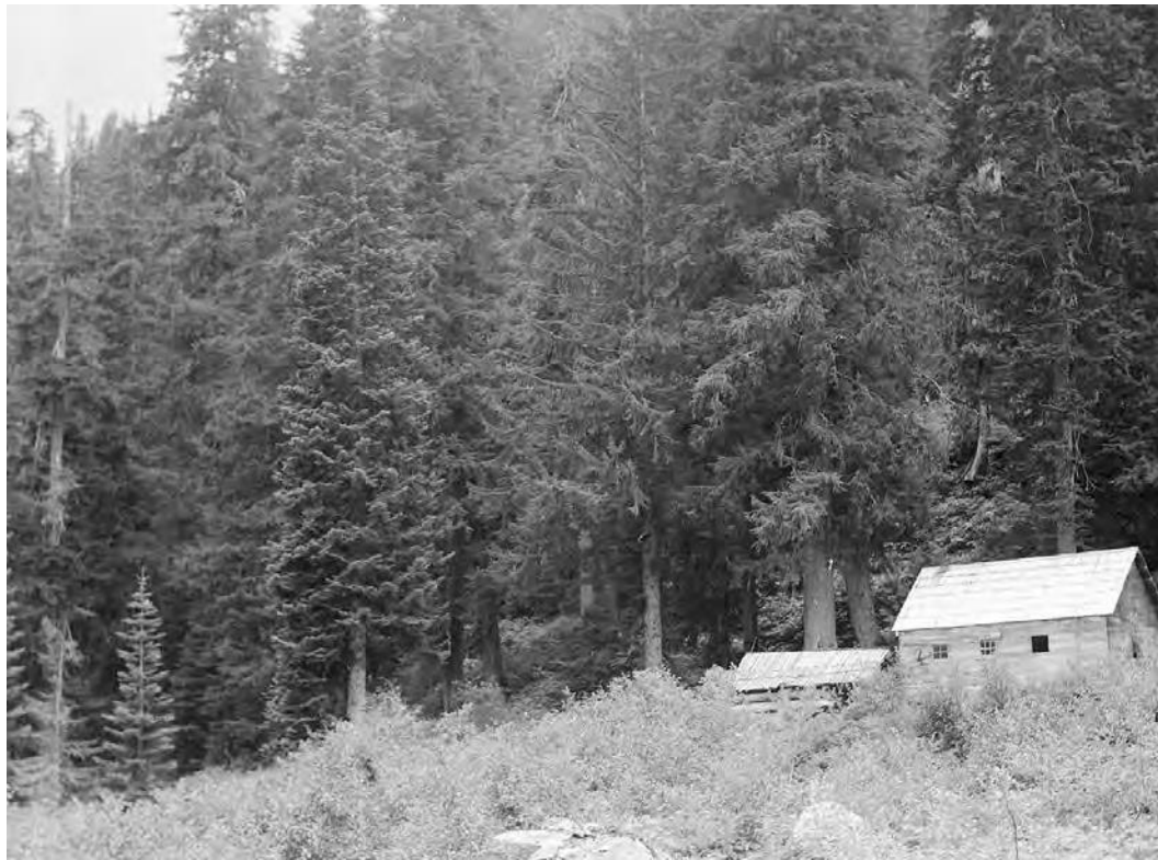
Figure 8: View down valley (i.e., southeast) of cabin on the Mineral Creek claim in 1945. Mineral Creek is to the left and the Mineral Creek Trail (#1331) to the right. The mill site is about 30 m further down valley and to the left (Panieri, 1945).
