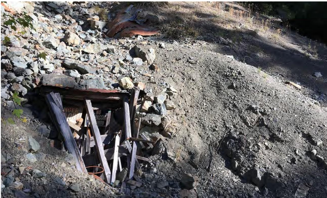
Figure 34: Partially sealed portal at the Maud O AML site. Photo taken looking north. The edge of the tailings pile can be seen to the right the portal. Photo by Scott Kugel, September 2017.
