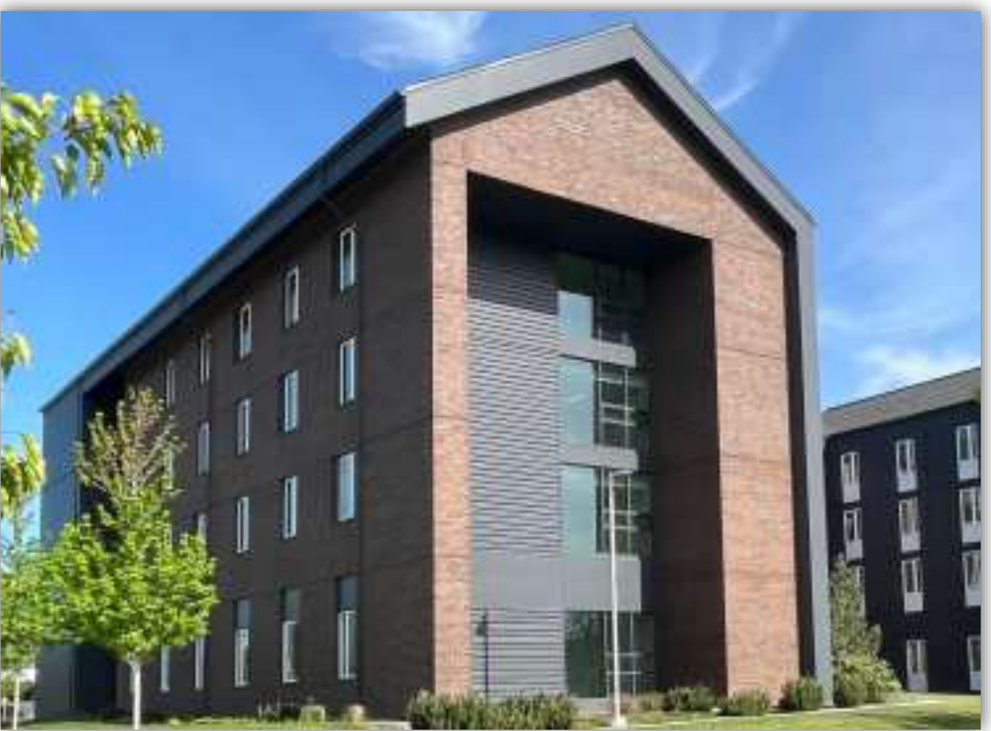
Figure 4. Picture of Dugmore hall
