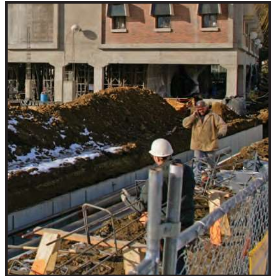
Work on “utilidors” near Dean Hall.
