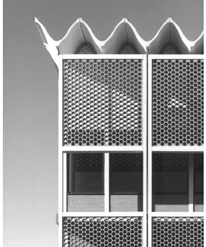
Unreinforced concrete & masonry exterior screens.
