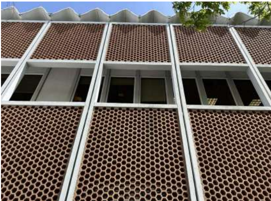
CWU Bouillon Hall - Existing Sunscreen
