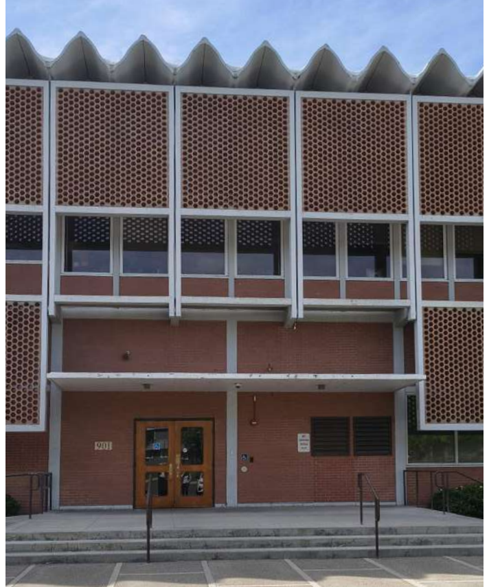
Uninviting east entry, converted from a former loading dock.
