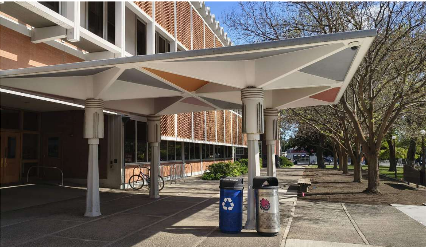
Bouillon Hall existing west campus-facing entry articulated with a dynamic and colorful concrete canopy.
