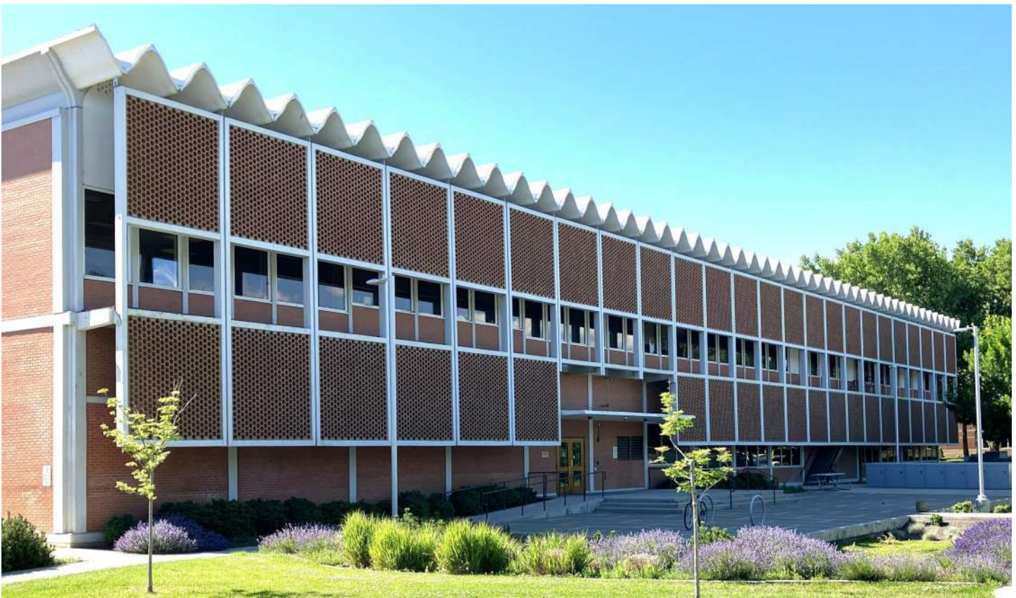
The east entry, former building service and loading point - now primary approach by vehicle for students and visitors, lacks the architectural prominence needed to welcome prospective students and guide them to the resources within.
