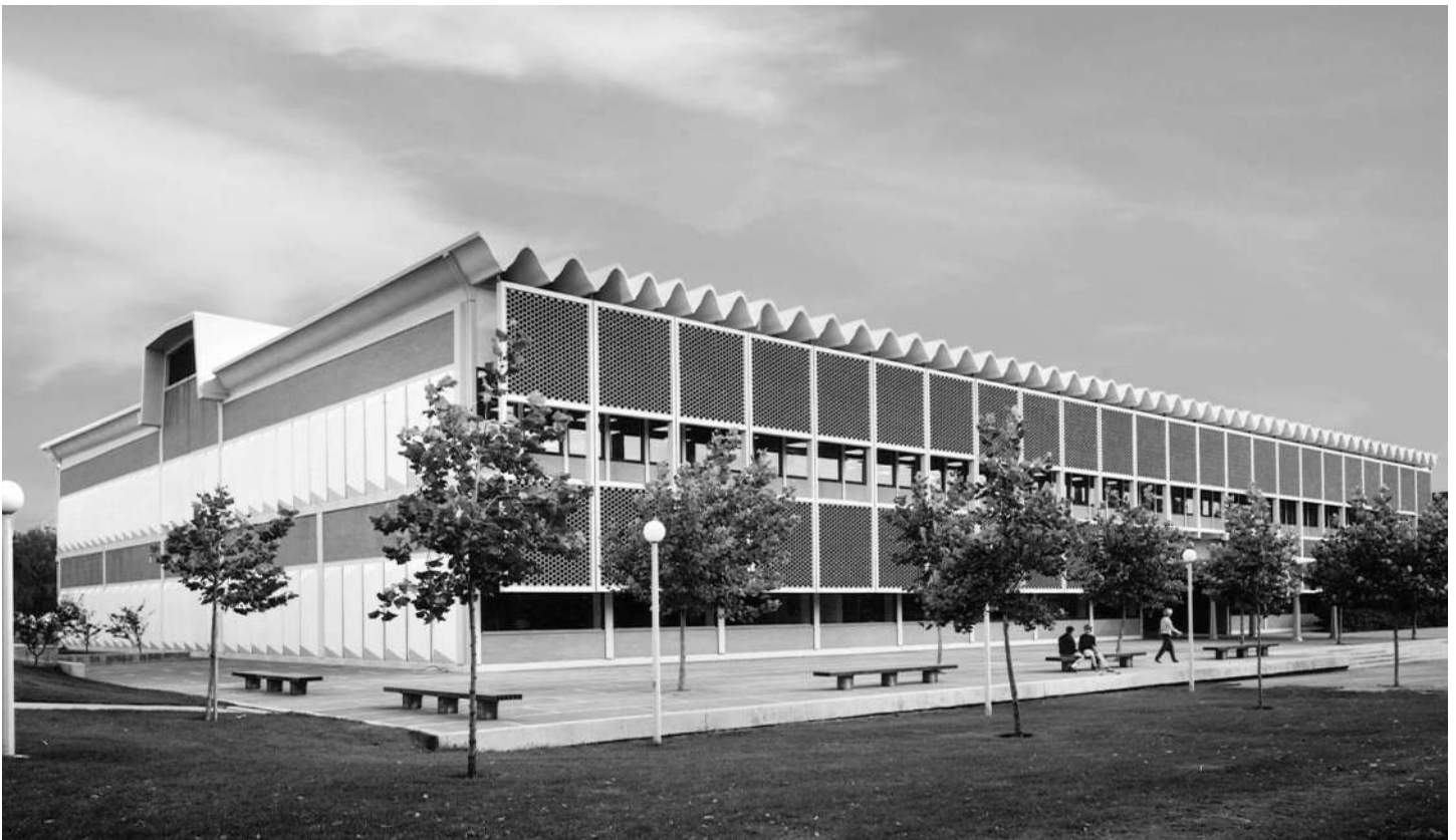
Character-defining mid-century features - specifically the faceted north facade, structural precast concrete folded roof plane, and unreinforced concrete/masonry screens - serve as a vital architectural anchor and visual gateway for the campus.
