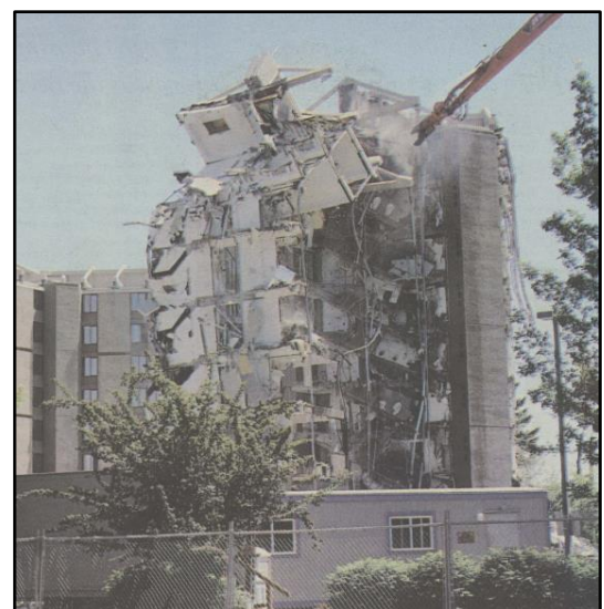
Courson Hall Demolition (The Observer, 2008)
